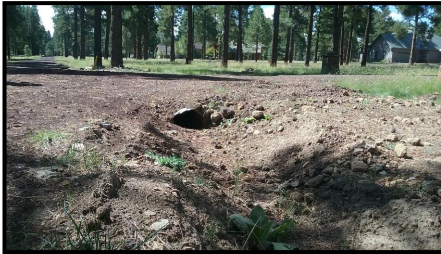
Figure 8: Existing Culvert, Photo by: McKenzie Moten [1]
