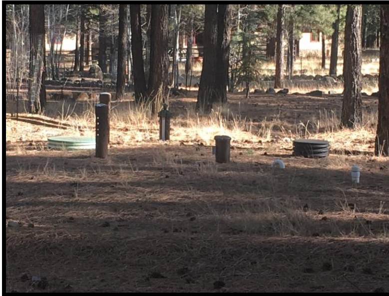
Figure 6: Existing Conditions- Well System, Photo taken by: McKenzie Moten [1]
